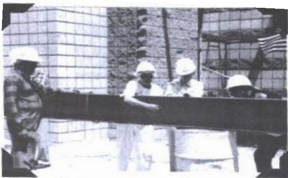
Signing the final beam for the Science Building are (from left) Tom Elder, Maxine Moore, Bettye Underhill and Dick Powell.
