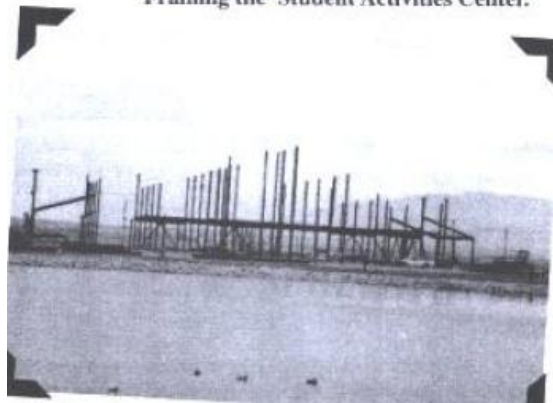
Framing the Student Activities Center.
